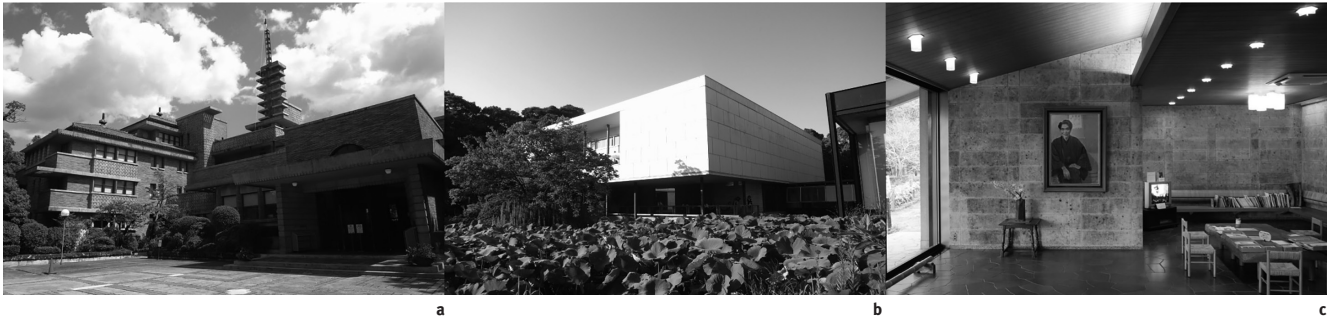
Fig. 3. Images of Arata Endo, Junzo Sakakura and Yoshiro Taniguchi's Works: a. Former Koshien Hotel; b. Former Kanagawa Prefectural Museum of Modern Art; c. Yoshikawa Eiji Museum© Akio Yasumori, 2019.
